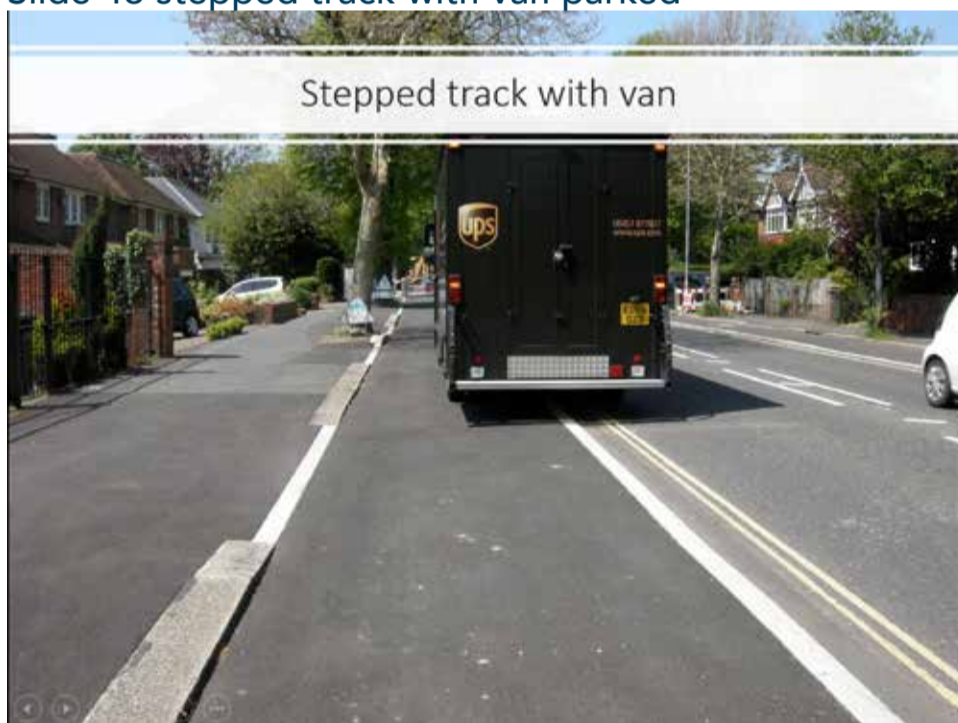
Slide 43 stepped track with van parked
